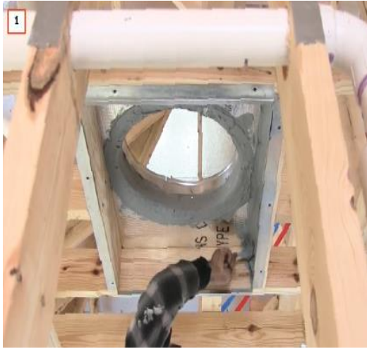
HVAC DUCT MASTIC -SEAL
