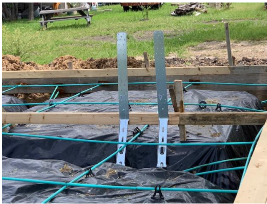
SIMPSON STRONG TIE – STHD-LSTHD-S INSTALLED AT FOUNDATION PRE-POUR
