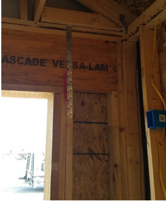
SIMPSON STRONG TIE – MSTC STRAP APPLIED TO A ROOM CORNER
